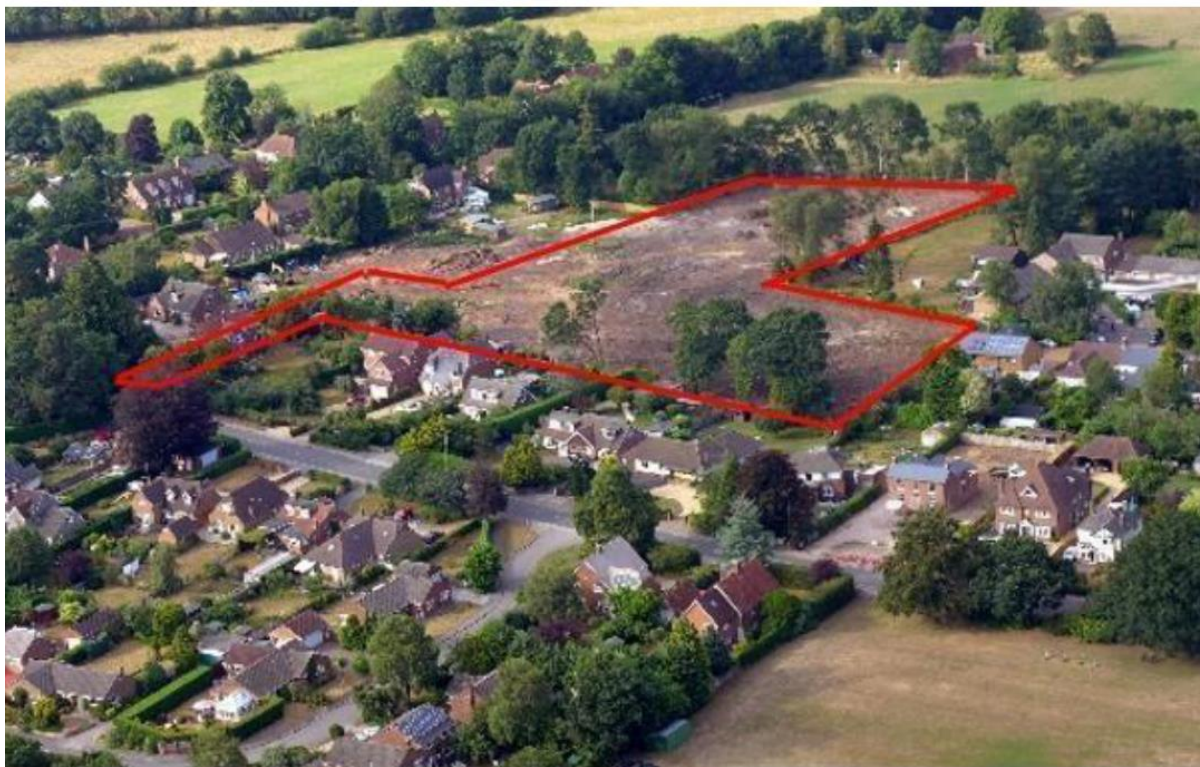
Aerial photo of application site with land to the west cleared prior to the construction of 5 dwellings now nearing completion.
